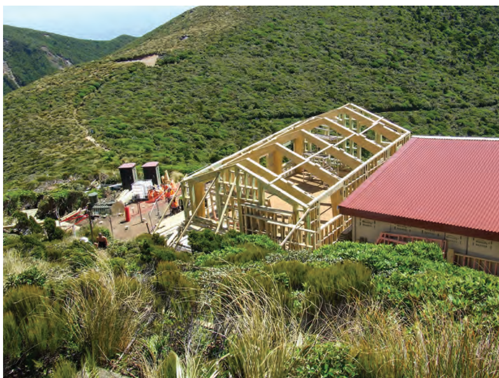
Extensive renovations to the Pouakai Hut being made.
